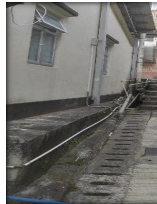
Congested space for utility work without proper clearance
