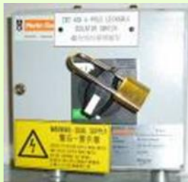
Lockable Isolation Switch
