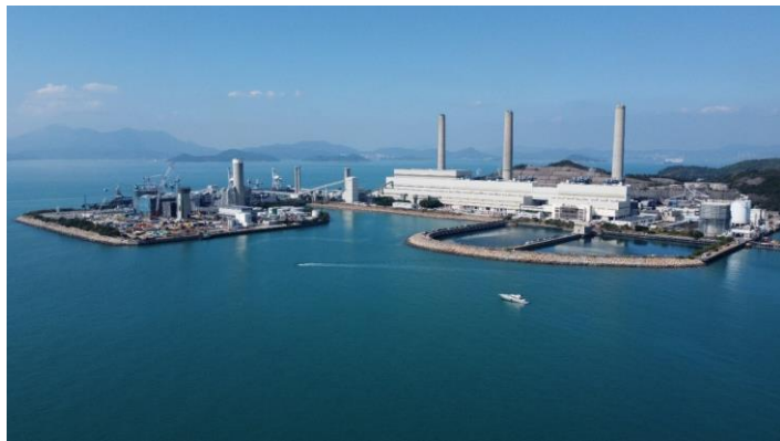
HKE - Lamma Power Station
