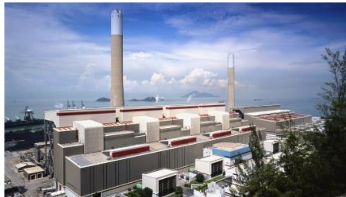
CLP - Castle Peak Power Station
