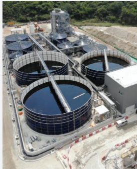
Using Landfill Gas for Ammonia Stripping
